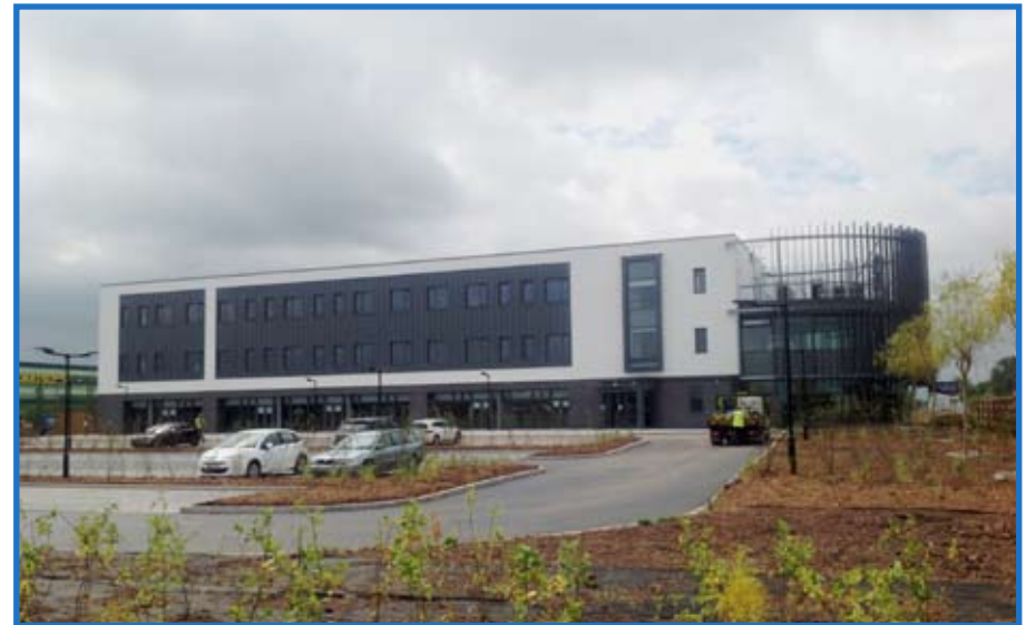
Bridgwater Enterprise and Innovation Centre
